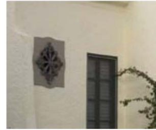
Cast Concrete (accent material)
