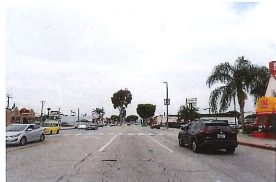
Photo 2: Existing conditions near Tyler Ave
