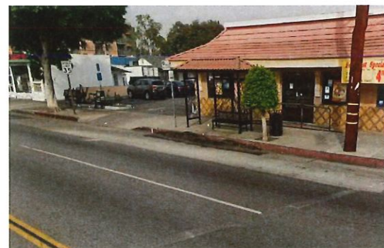
Photo 9: Bus pullout with shelter
