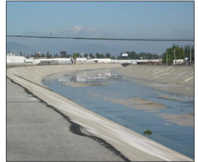
Flood Control Channels
