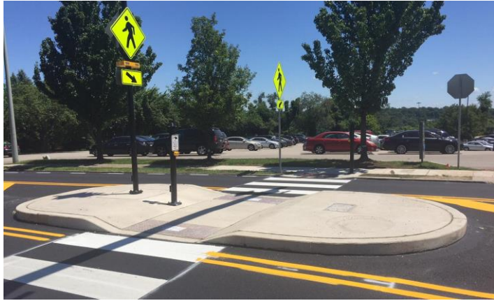
Pedestrian Refuge and Rectangular Rapid Flashing Beacon
