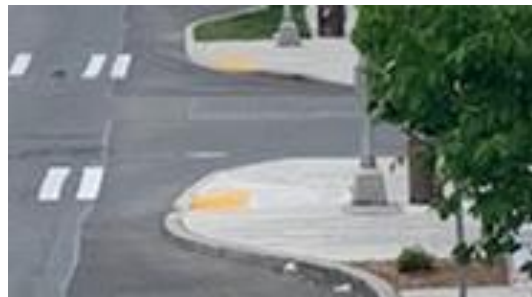
Concrete Bulb Outs
