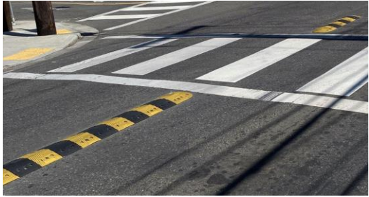
Hardened Centerline and High Visibility Crosswalks
