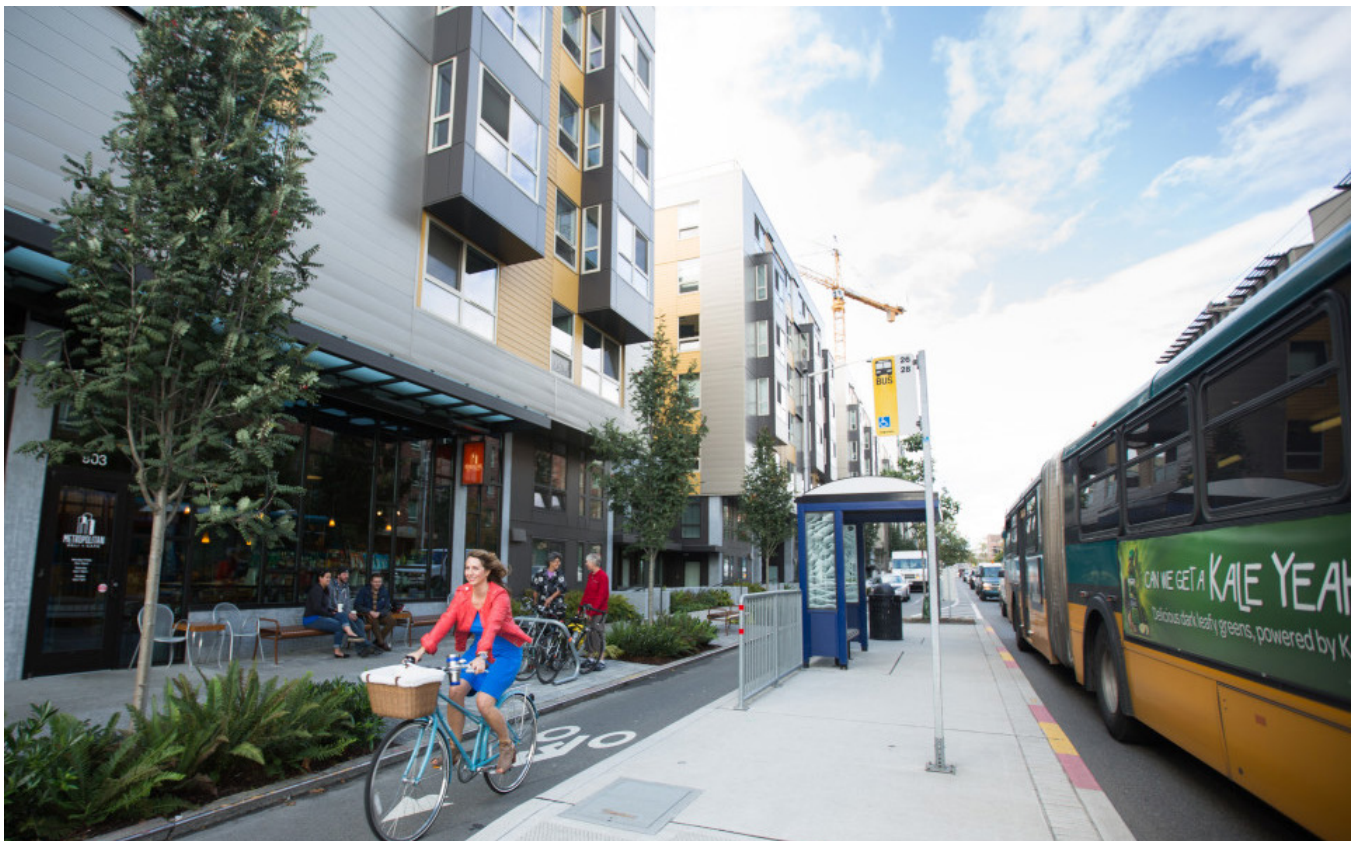
A bus separated bikeway (Class IV) and Bus Boarding Island separate user modes and enhance the multimodality of the street
