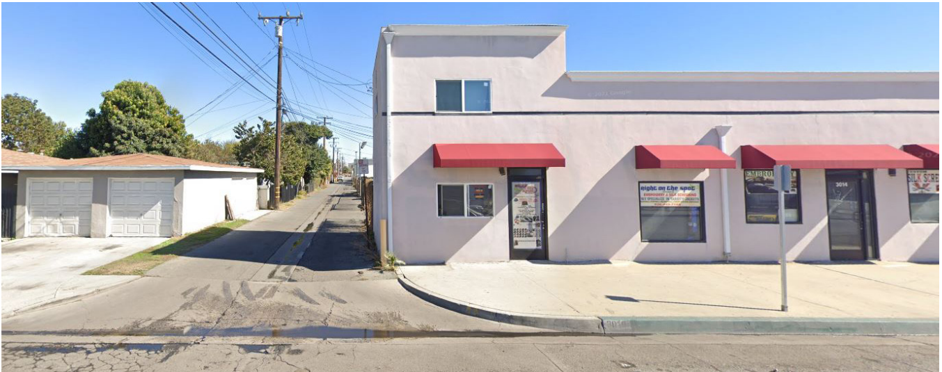
C - Urban Service Alleyway - the Paseo North of Garvey viewed from Consol Avenue
