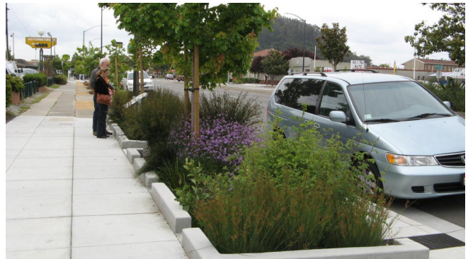
Stormwater receptive planting captures water from roadway
