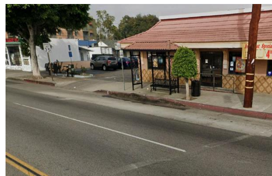
Photo 9: Bus pullout with shelter
